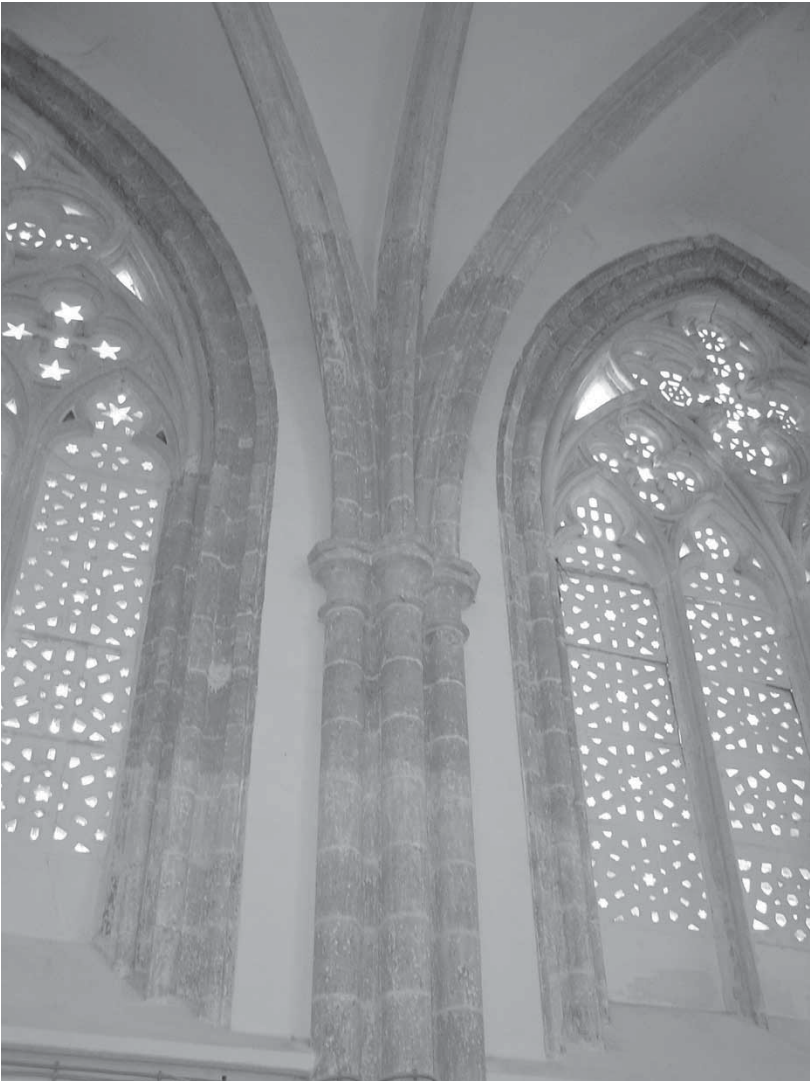
Fig. 43: Famagusta Cathedral, nave, wall respond [M. Olympios].
